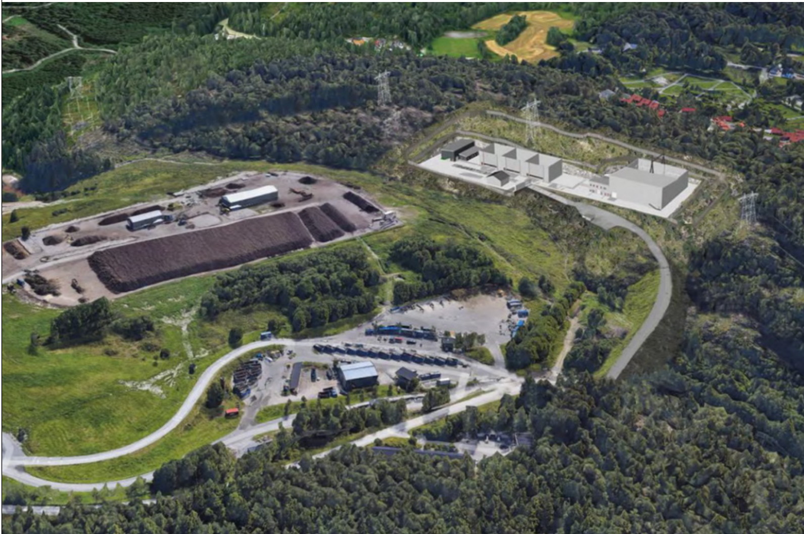
Liåsen transformer station - detail design, Norway | Photo: Statnett
