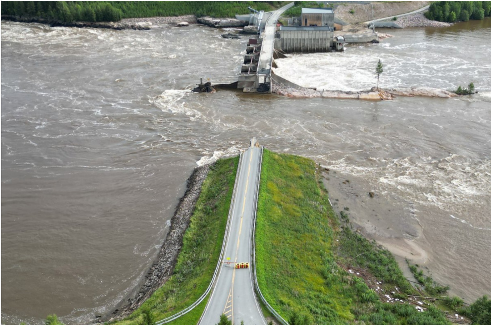
Reconstruction of the Braskereidfoss dam Norway | Photo: Hafslund
