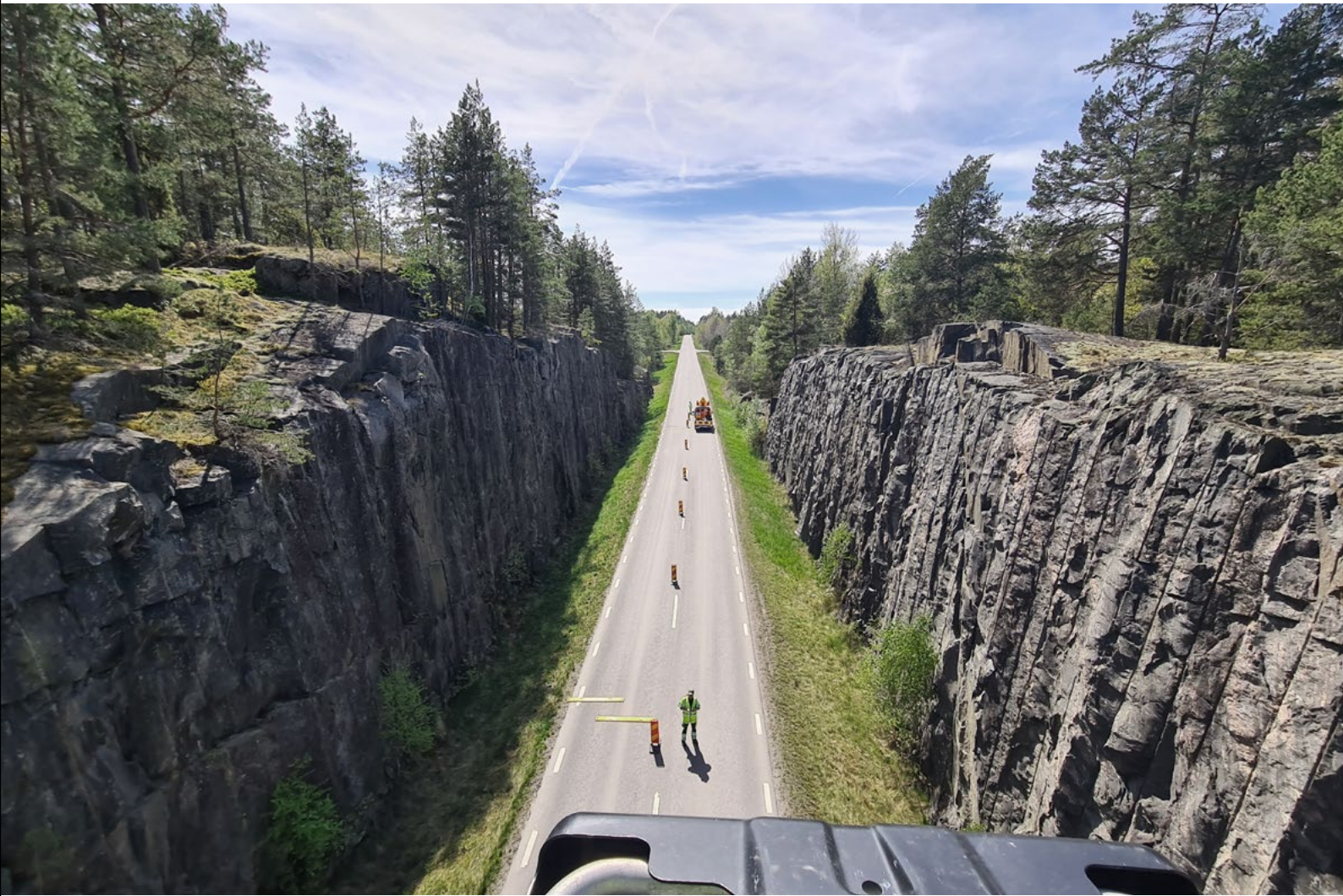
Inspection of road cuttings in Västra and Värmland County, Sweden | Photo: Norconsult
